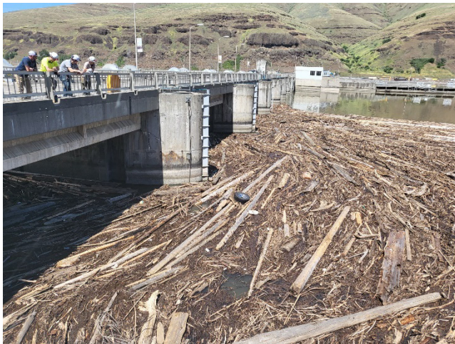
LWG forebay debris June 15, 2022.
